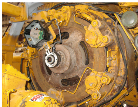
Encoder, gearbox and motor ready for final assembly
